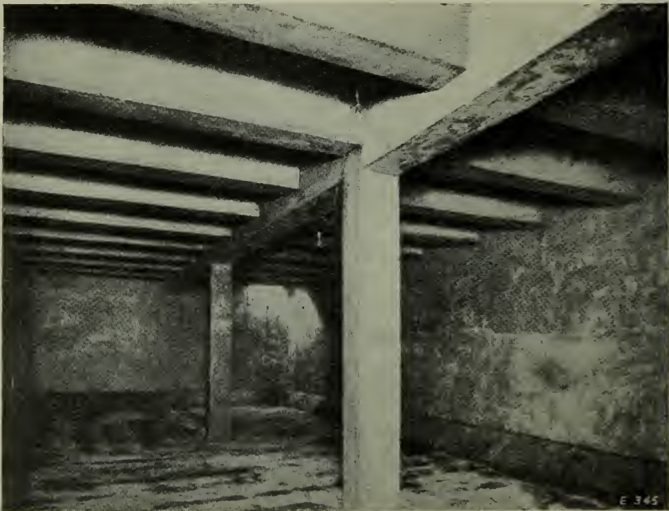
INTERIOR VIEW OF 150,000-GALLON CONCRETE OIL TANK.
